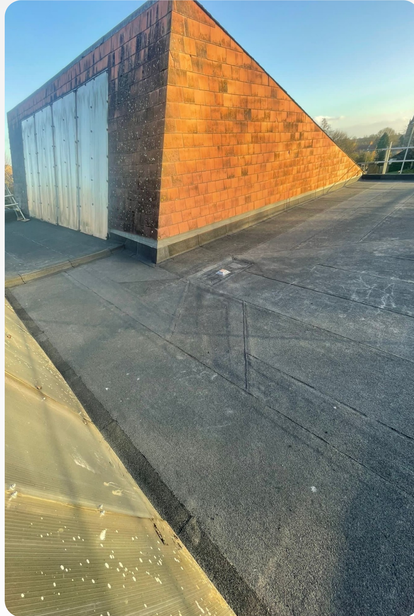
Above After works
