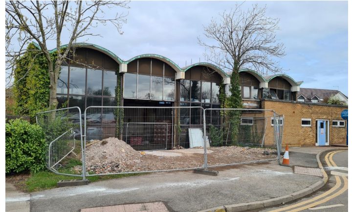
Front elevation: prior to roofing works
