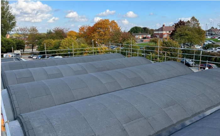
Roof A: Completed barrel roof
