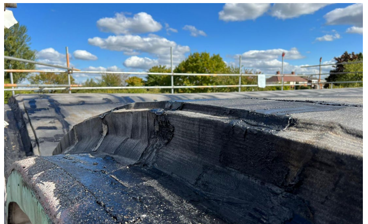
Roof A: Interim inspection of newly installed timber hard edge
