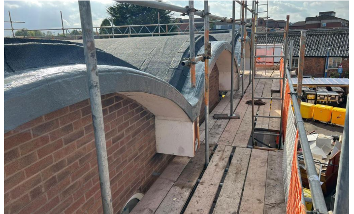
Roof A: Completed application of PMMA to the existing copper fascia
