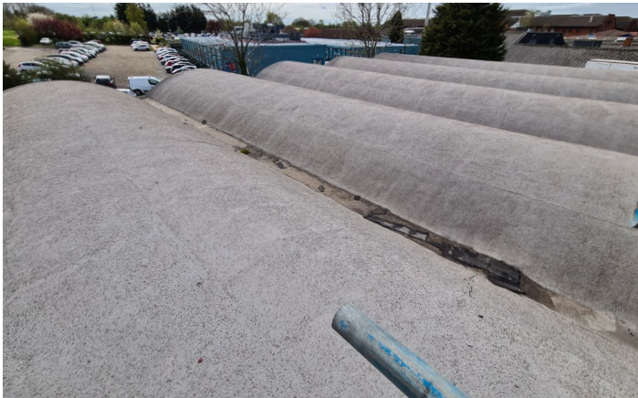
Roof A: Original uninsulated barrel roof with asphalt finish
